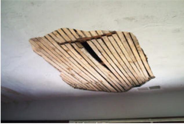
This is a recent ceiling repair that I did. This old damage from a leaking roof that was repaired but the hole in the ceiling was never touched. I also removed any debris from the attic above.
