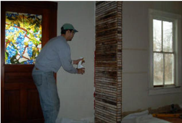
Preparing for the first layer of plaster (the scratch coat), I lightly spray the dry lath with water just before applying the scratch coat. This prevents cracking due to rapid absorption from the dried out wood lath.
