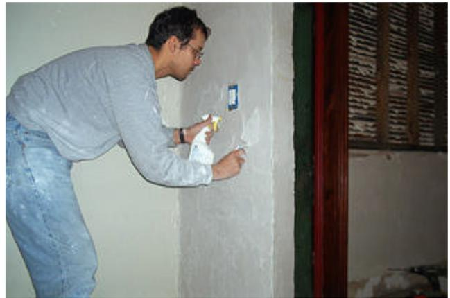
The second coat, the brown coat, is not shown but it looks similar to the scratch coat, just 3/8 inch thicker. Here I am putting the final layer of plaster on the arch. I will smooth it out by spraying it with water while it hardens.
