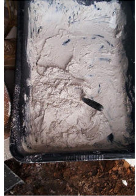
Shown in the left photograph are equal piles of Diamond Plaster (on top) and the Structo- on the bottom scooped into a large cement trough. In the middle photograph, the two plasters are dry-mixed together and any hard lumps are crushed into powder. Remove any lumps larger than a dime and discard them as too many will cause the mixture to set too rapidly. Mix with enough enough water to create the consistency of cake batter but just a tad soupy. The extra water increases the working time.
