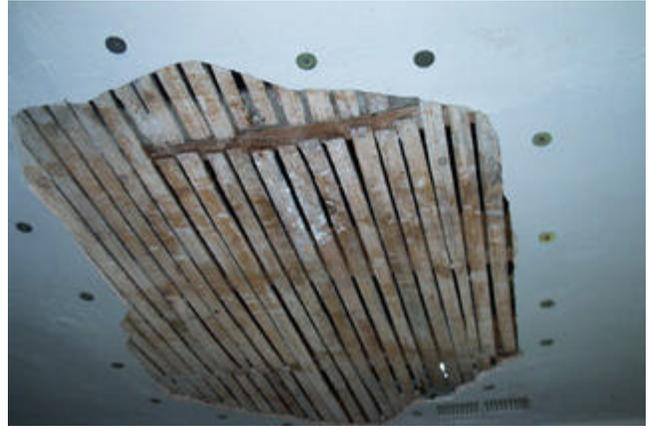
Due to some warping in the wood, I reattached the lath using screws. I then used drywall screws and fender washers to secure the old plaster better to the wood lath.
